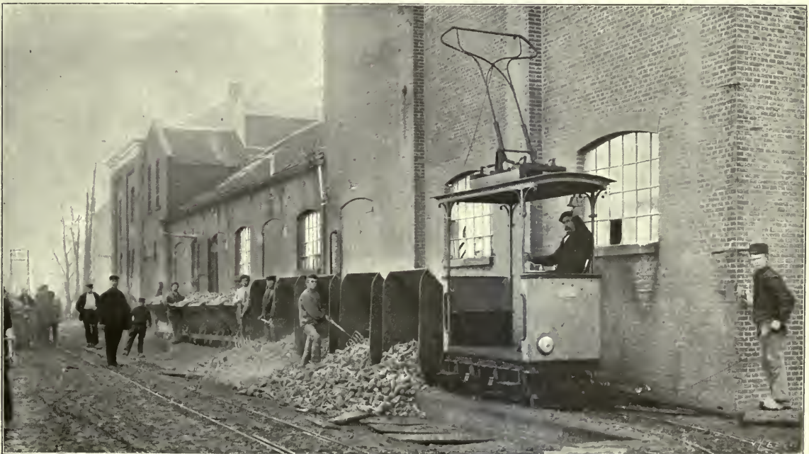
TRANSPORTING BEETROOTS TO THE FACTORY BY AN ELECTRIC TRAIN
