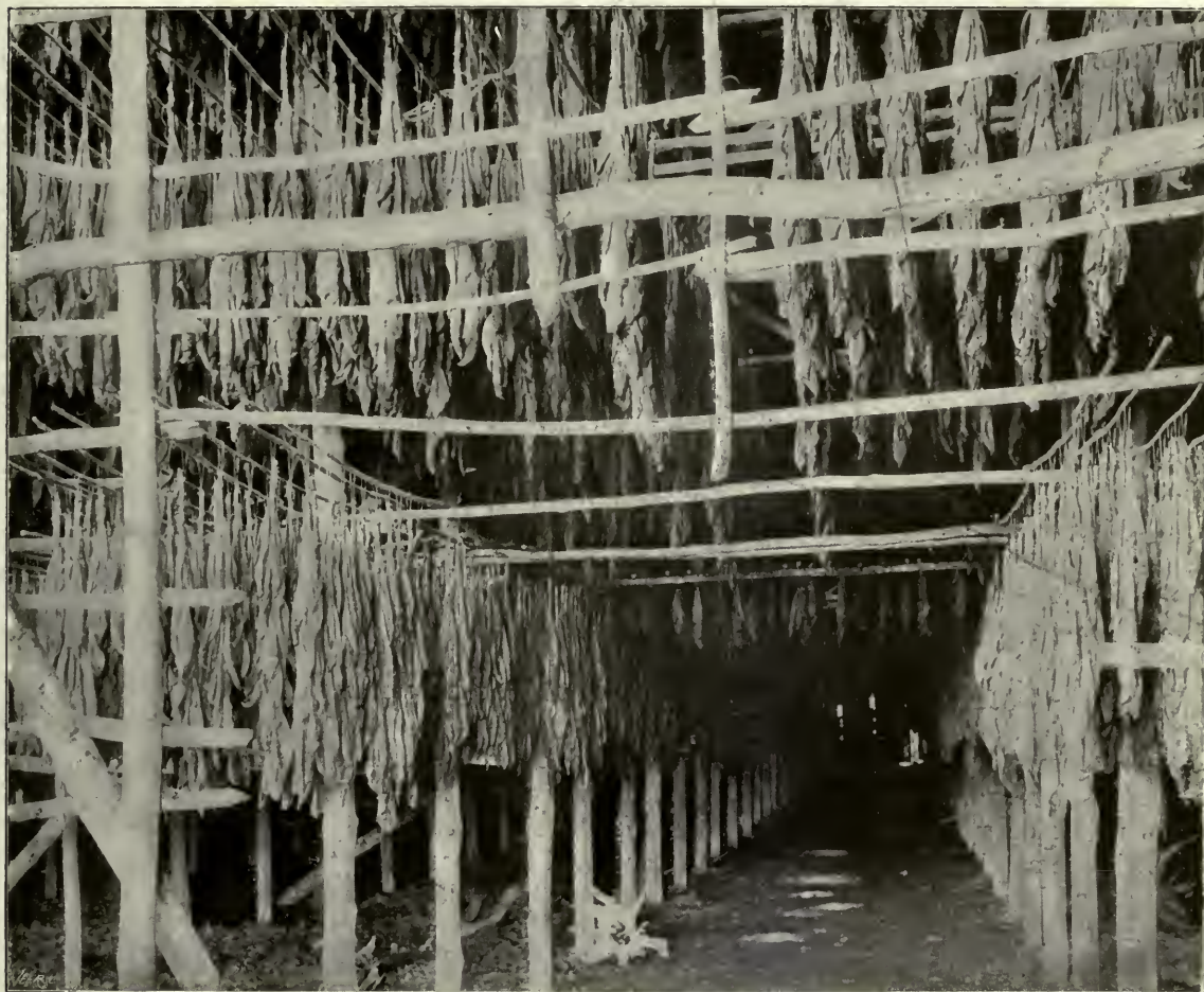
THE INTERIOR OF A CURING BARN
