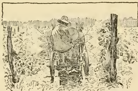
Fig. 67. Two-horse spray machine for grapes.
