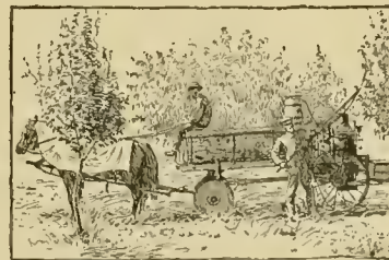
Fig. 70. Spray rig with steam power pump.
