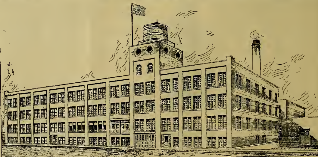
The New Manufacturing and Milling Plant of the Foley Manufacturing Company, Chicago
