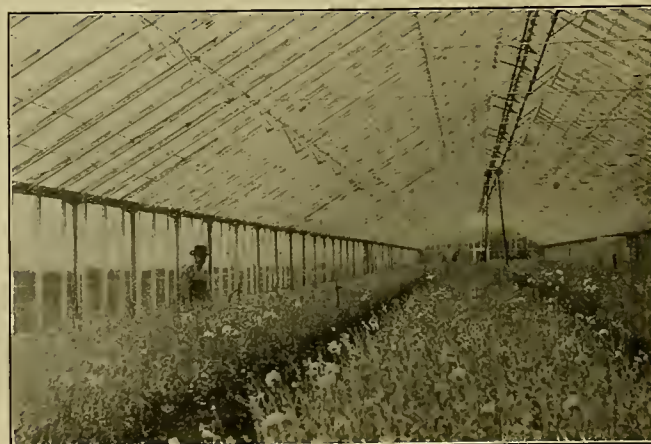
Coles's King Construction Carnation House
