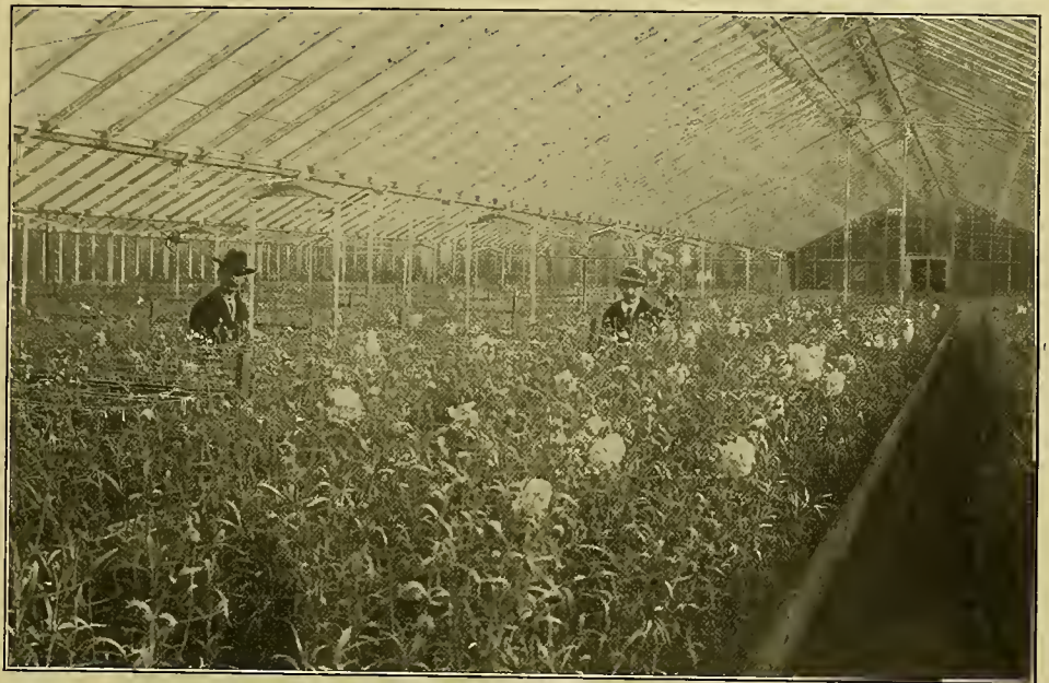
New Greenhouse (King Construction) Rose Hill Greenhouses, Columbia, S. C.
