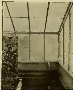
The way interior of a steel eave house looks
