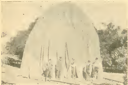
FIG. 2.—Tent in position for fumigation.
