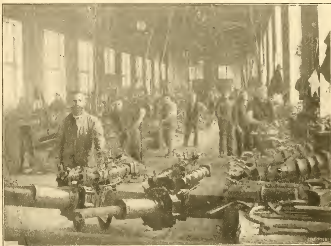
FIG. 1.—Workshop in Brieg, Switzerland, at the foot of the road leading over the Simplon Pass. In the foreground are two boring chisels mounted on one stand. (From Die Umschau .)
