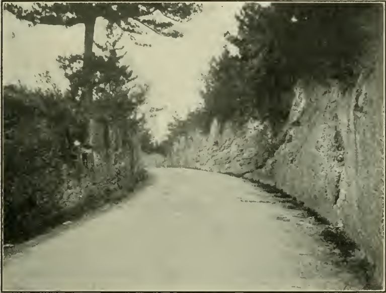
Figure 12.—Road Cutting near Hamilton.
