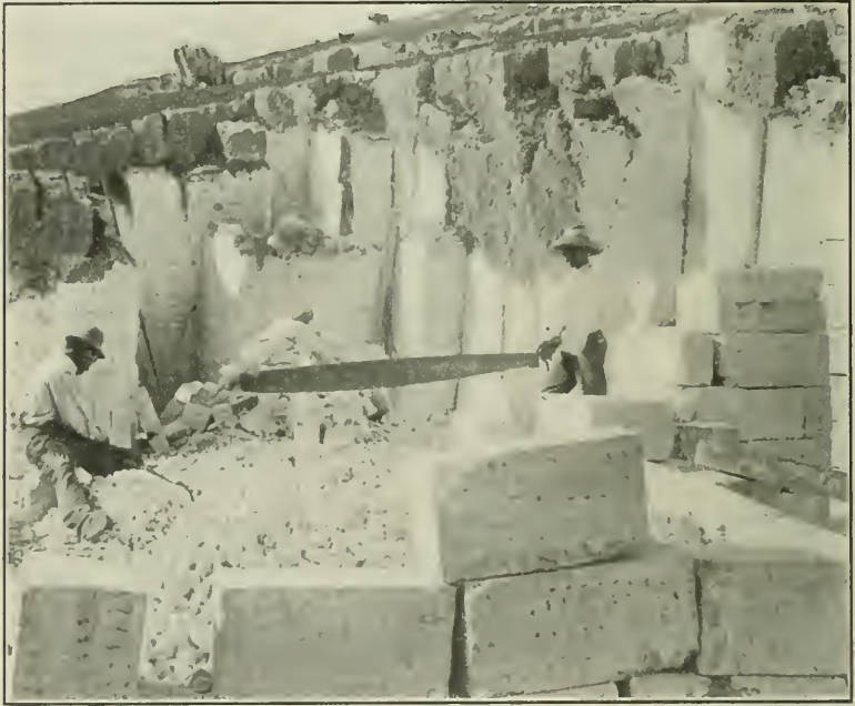
Figure 11.—Quarrying Limestone with ehisels and saws.
