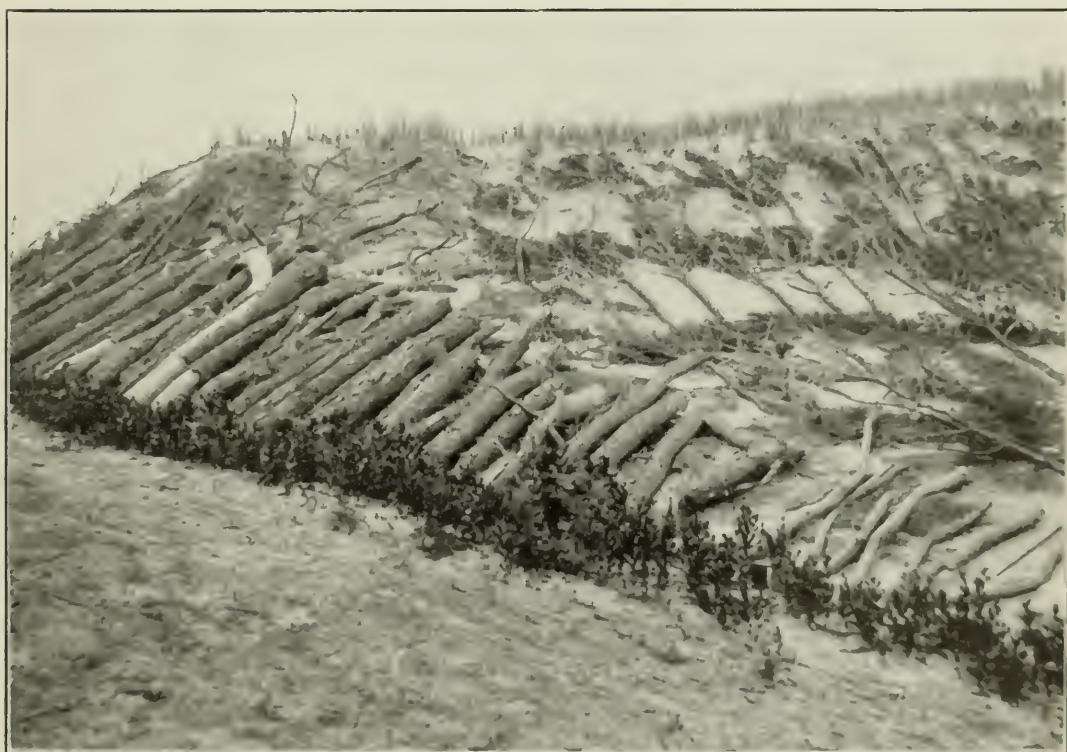
FIG. 2.—PROTECTING A ROAD THROUGH THE DUNES.
