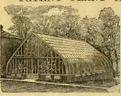
CURVILINEAR SPAN-ROOF HOUSE.
