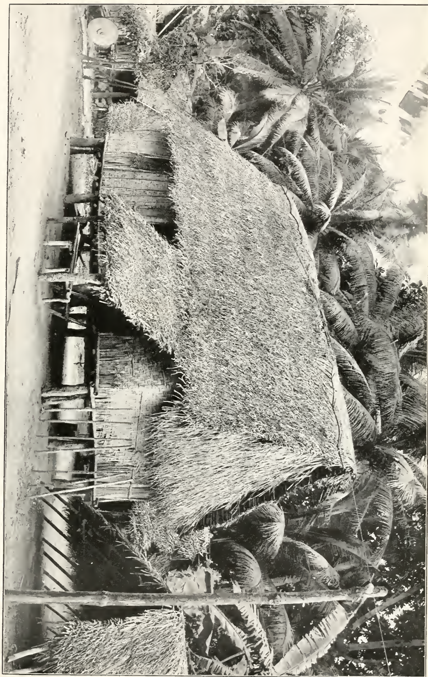
TYPICAL NATIVE DWELLING, ISLAND OF GUAM. SIDES OF BAMBOO AND WOVEN REEDS AND ROOF OF COCONUT THATCH.
