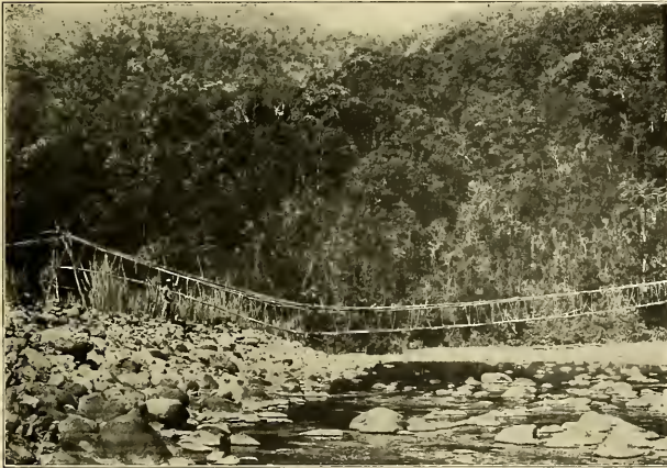
Fig. 2. Rattan bridge built by Mangyans, near Sablayan.
