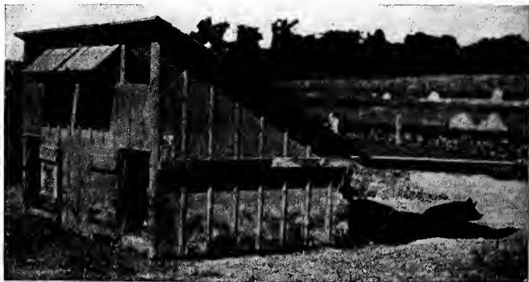
FIG. 83.—Portable hog-houses with low, flat roof; if used for housing swine in hot weather, they should be provided with a shade at the rear under which the pigs can lie in comfort. This shade is five feet wide, made of inch stuff placed upon removable supports which rest upon cleats nailed to the ends of the house. (Wisconsin Station.)
