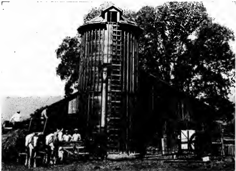
FIG. 30.—A “re-saw” silo being filled with alfalfa. These silos are well adapted to mild climates, as that of California and the southern States. ( Pacific Rural Press. )
