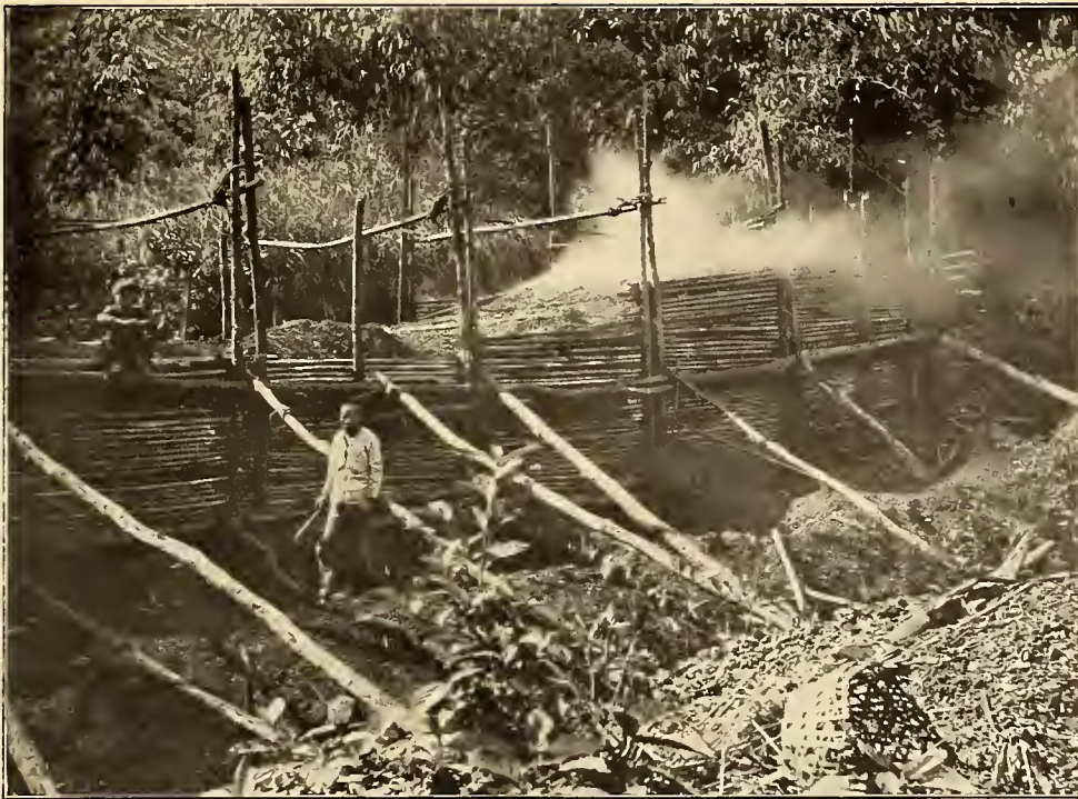
Fig. 1. Charcoal burning; wood in place in kiln.
