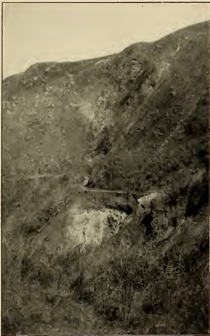
PLATE VI. OLD SPANISH ROAD TO COPPER MINES, MANCAYAN, SHOWING CONTACT BETWEEN OVERLYING QUARTZ PORPHYRY AND MANCAYAN DIORITE.
