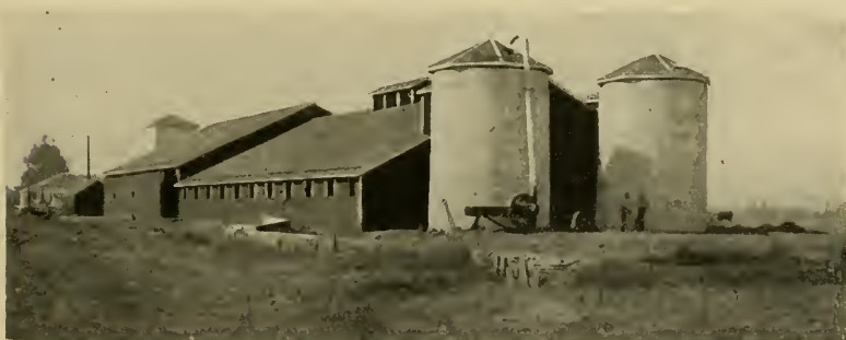
FIG. 29.—A California dairy barn, with concrete silos, accommodating four rows of cows, with a driveway in the middle.
