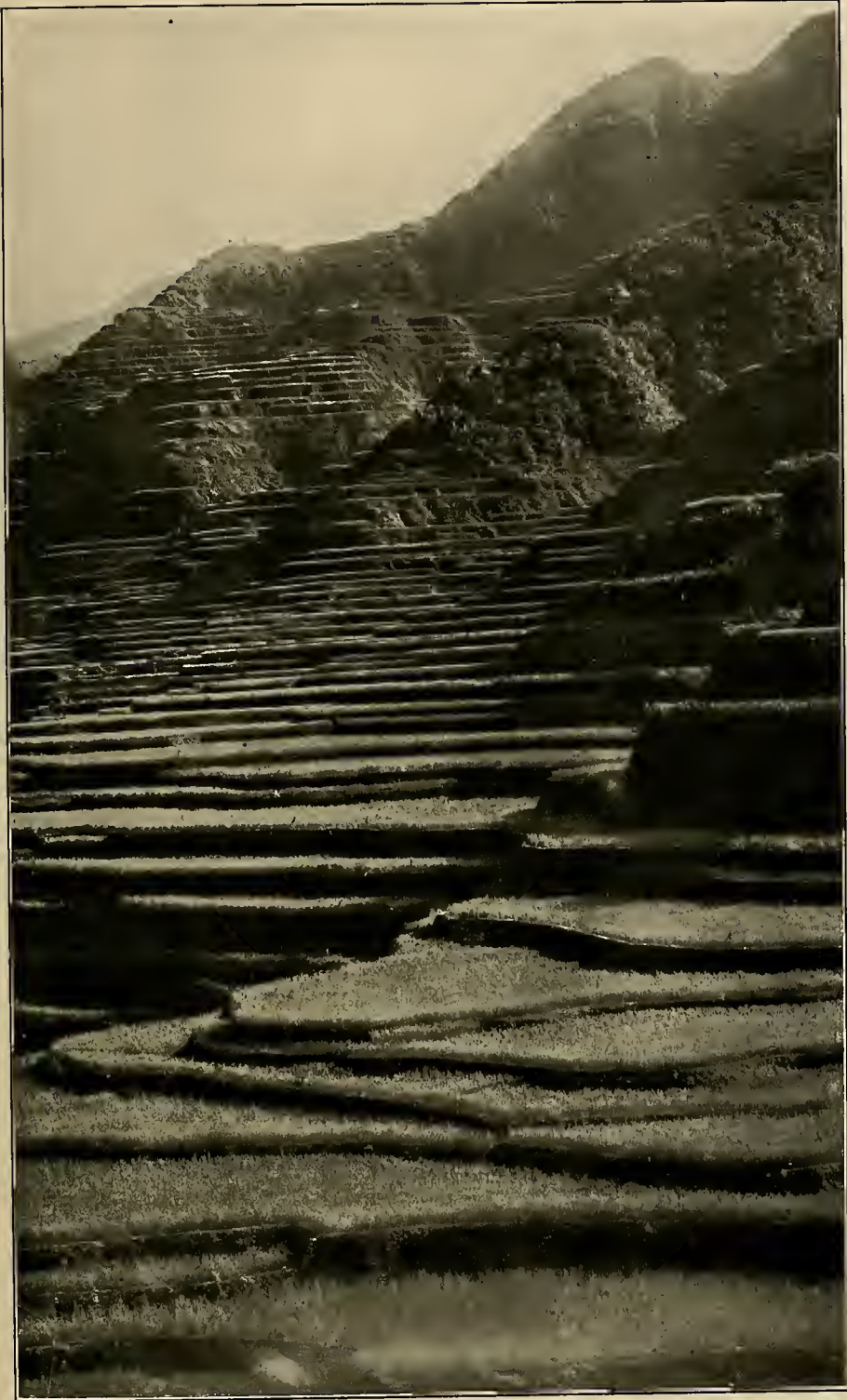
IFUGAO RICE TERRACES WITH STONE RETAINING WALLS, BANAUE.
