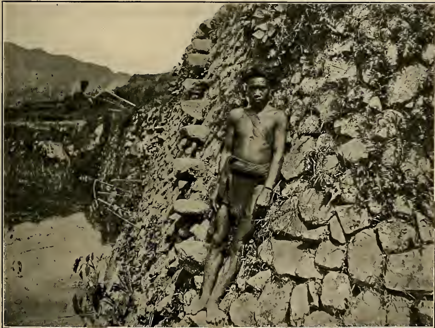
FIG. 2. STONE RETAINING WALL OR "PILAPIL" WITH PROJECTING STEPS.
