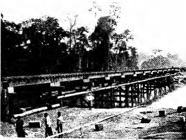
FIG. 99.—The temporary Wooden Bridge over the Imo, on the Eastern Division, Nigerian Railway. Note, only native, locally grown timber used in its construction.
