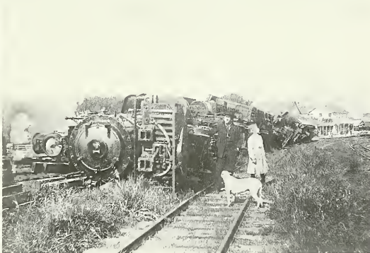
FIGURE 28. Point Reyes Station. Train overturned by the earthquake. G.K. Gilbert photograph [GKG 3400]. U.S. Geological Survey Photographic Archives, Denver, Colorado.
