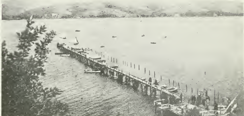
FIGURE 15. Bailey's Pier at Inverness. Photo taken by Martha P. Schreiber before 18 April 1906 (from Gilbert in Lawson, 1908, pl. 58, fig. B).
