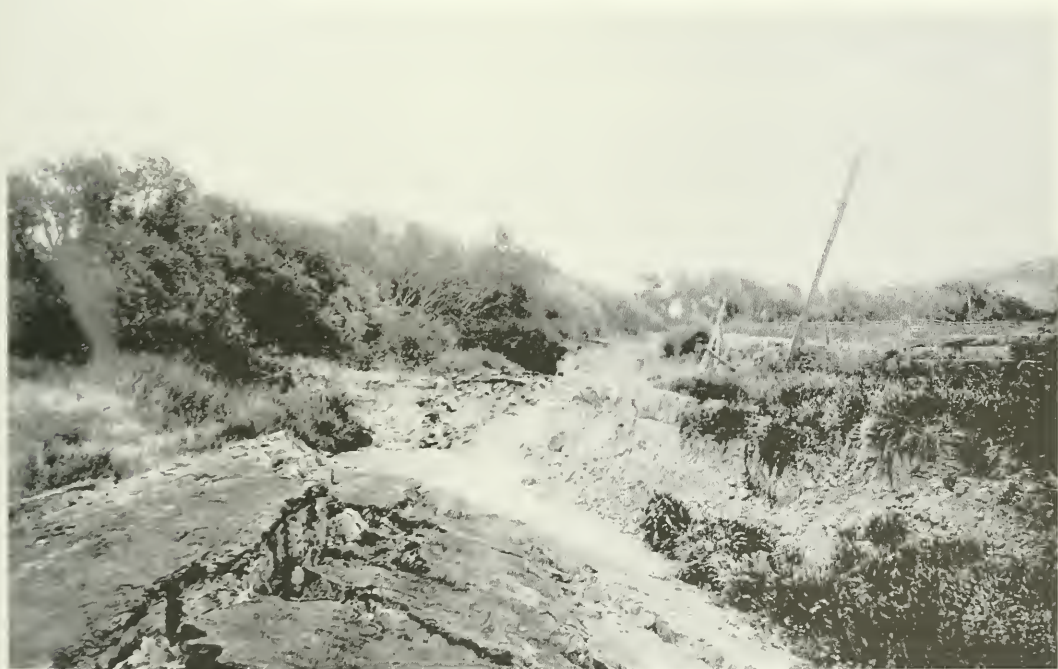
FIGURE 12. Road bed between Olema and Inverness. Road bed probably destroyed by shaking of soft ground beneath. Photograph by G.K. Gilbert. (G.K. Gilbert Collection [N-7583-F], California Academy of Sciences Archives.)
