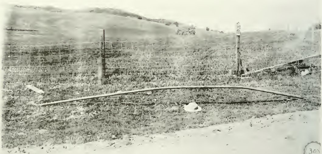
FIGURE 14. Buried water pipe upended by earthquake motion. Five miles west of Stanford University along Portola Valley Road. Although among the Gilbert images, we suspect that this one was taken by John Branner, or a Branner student at Stanford University, and given to Gilbert. (G.K. Gilbert Collection [N7583-B], California Academy of Sciences Archives.)
