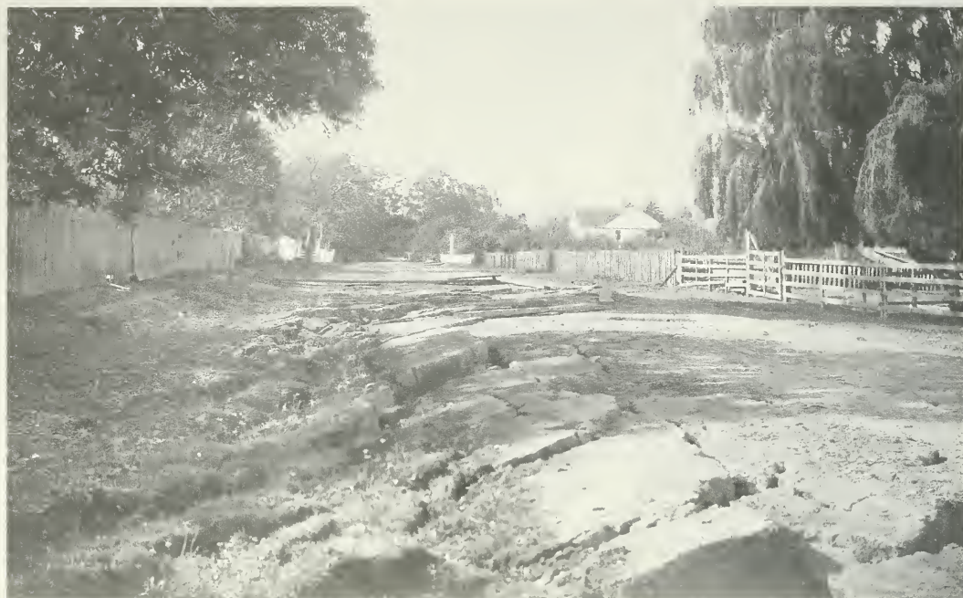
FIGURE 21. Branch of fault-trace in north part of Bolinas, looking NNW, illustrating diagonal cracks. Photograph by G.K. Gilbert. (G.K. Gilbert Collection [331.6.1, #165; Unnumbered white envelope], Alice Eastwood Archive, California Academy of Sciences Archives.) (Also in Gilbert in Lawson 1908, pl. 39, fig. A).
