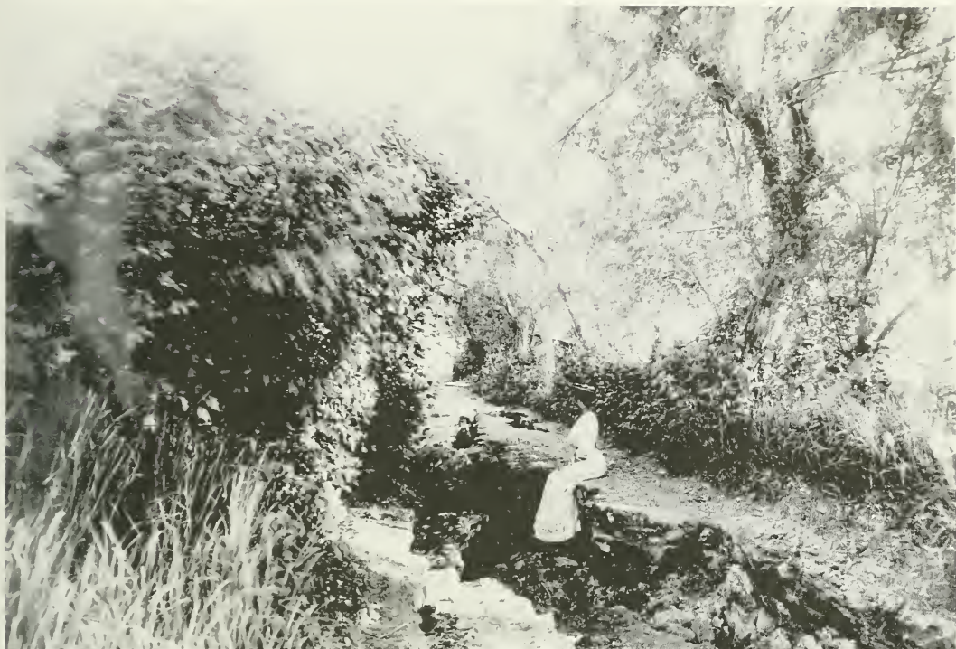
FIGURE 11. Road bed between Olema and Inverness. Collapse of road bed gives appearance of a vertical displacement about 5 feet. Photograph by G.K. Gilbert. (G.K. Gilbert Collection [N7583-E], California Academy of Sciences Archives.)
