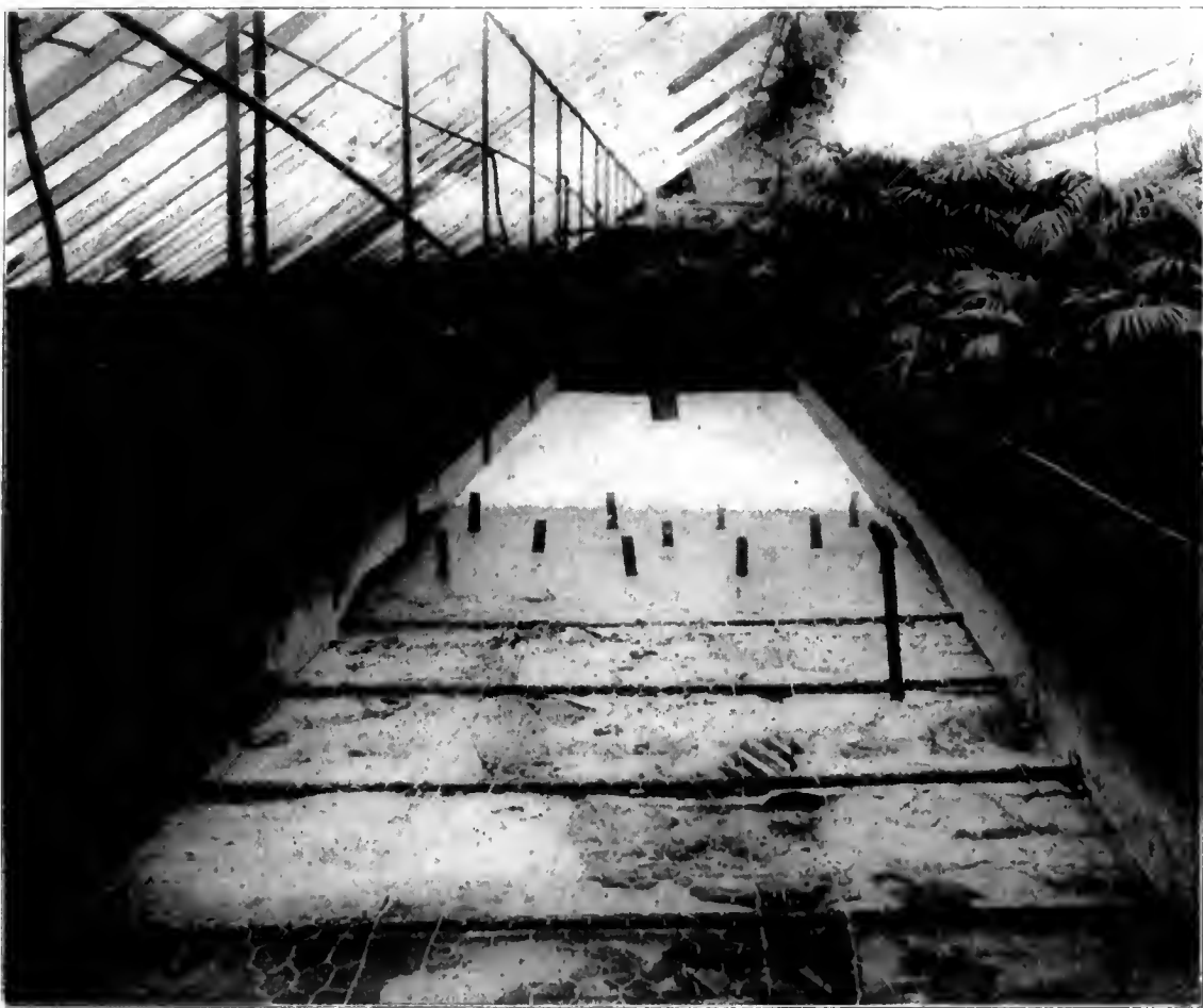
Cement Bench in Course of Construction at Wittbold's, Chicago.
