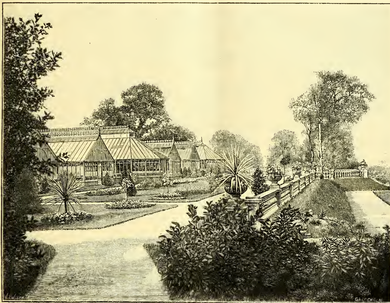
FIG. 8.—VIEW OF THE PLANT-HOUSES AT FAIRLAND PARK, NORWOOD. (SEE P. 39.)
