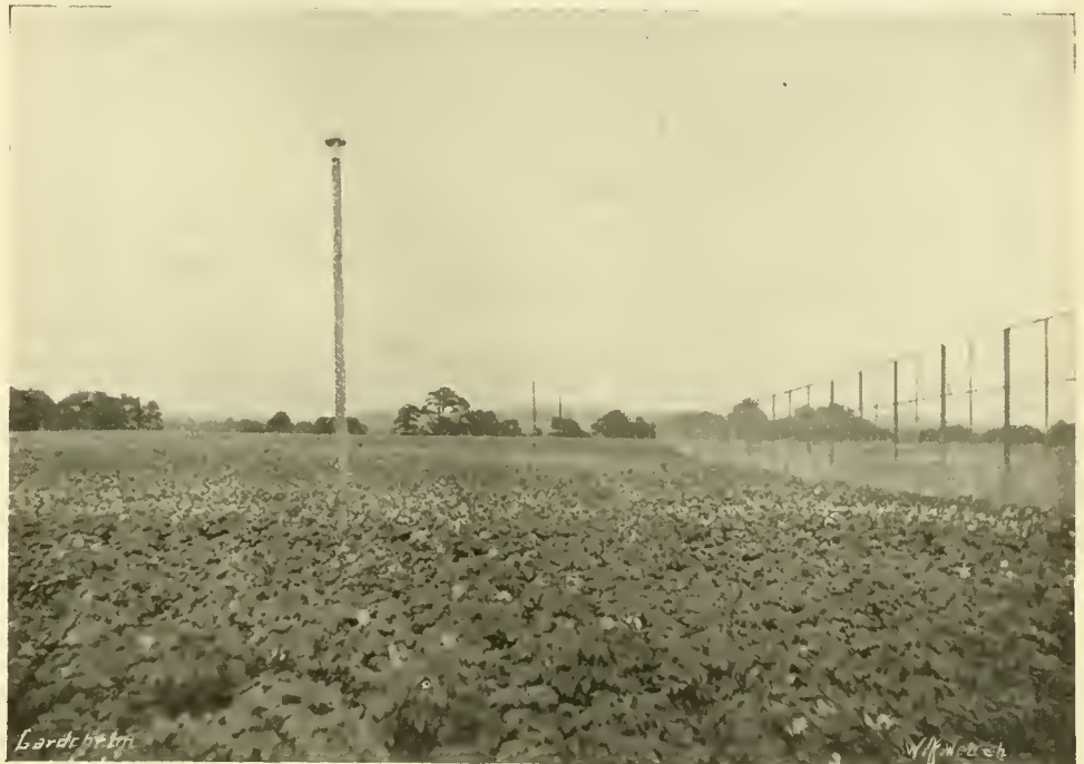
FIG. 107.—ELECTRIFIED AREA, DUMFRIES, 1913. LARCH POLES WITH INSULATORS SEEN IN THE CENTRE: THESE CARRY CHARGED OVERHEAD WIRES. ON RIGHT, WIRE NETTING ERECTED IN ORDER TO SCREEN THE CONTROL AREA.
