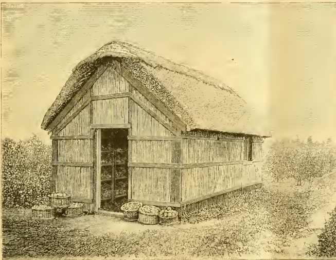
FIG. 113.—MESSRS. BUNYARD'S FRUIT-ROOM: WALLS OF REED, ROOF THATCHED.
