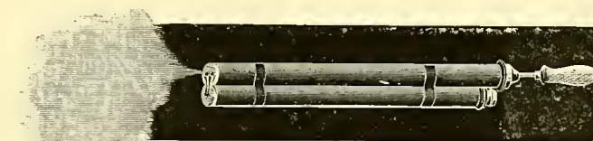
FIG. 16.—MR. C. E. WEST'S DOUBLE-BARRELLED SPRAYING SYRINGE, FOR EMPLOYING INSECTICIDES AND MIXING THEM WITH WATER.
