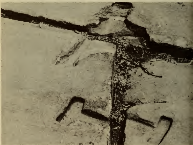
[20] Typical wall construction and detail of sockets for cast copper cramps or tie bolts in stone paving at Tiahuanaco.
