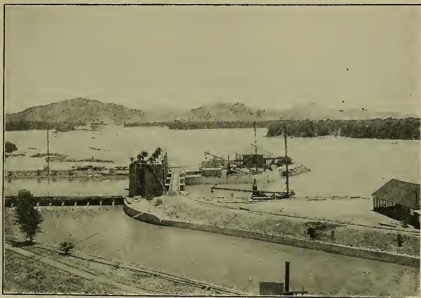
2. LAGUNA DAM, YUMA PROJECT.
