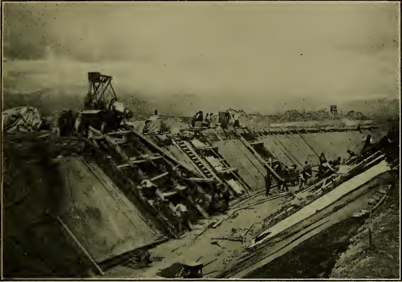
1. PLACING CONCRETE LINING, SUN RIVER SLOPE CANAL, SUN RIVER PROJECT.
