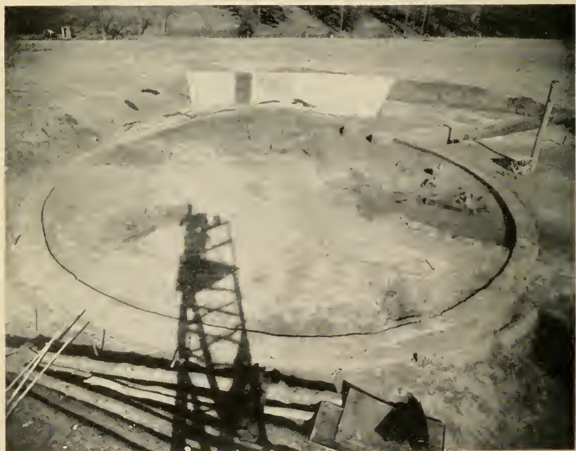
b , Beginning exploration to uncover floor of ceremonial earth lodge near Mound D, North (Macon) Plateau. The entrance passage, U-shaped clay buttresses in the entrance, inner fired clay wall periphery, debris of charred supporting timbers, and collapsed clay roof mantle arc features exhibited at this stage.
