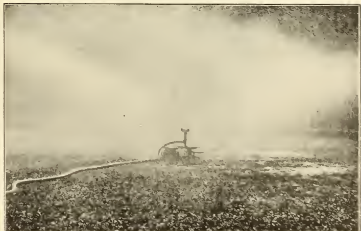
The Park Sprinkler.
