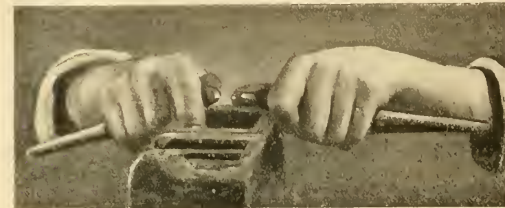
FIG. 2.—Diamond Bruting. From 'The Gem-Cutter's Craft.'
