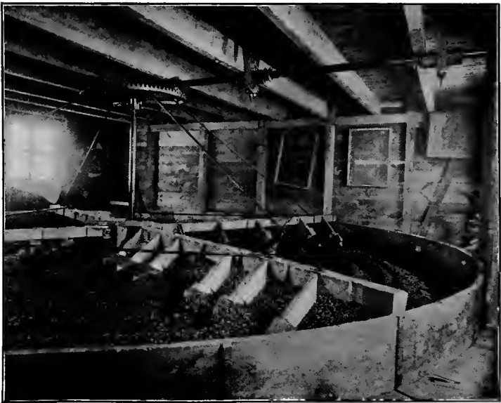
FIG. 51. HOADLEY'S KILN DRYER
