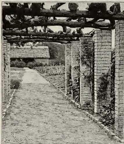
NEWLY-FORMED PERGOLA AT MUNSTEAD, WITH BRICK PILLARS AND OAK TIMBERS.
