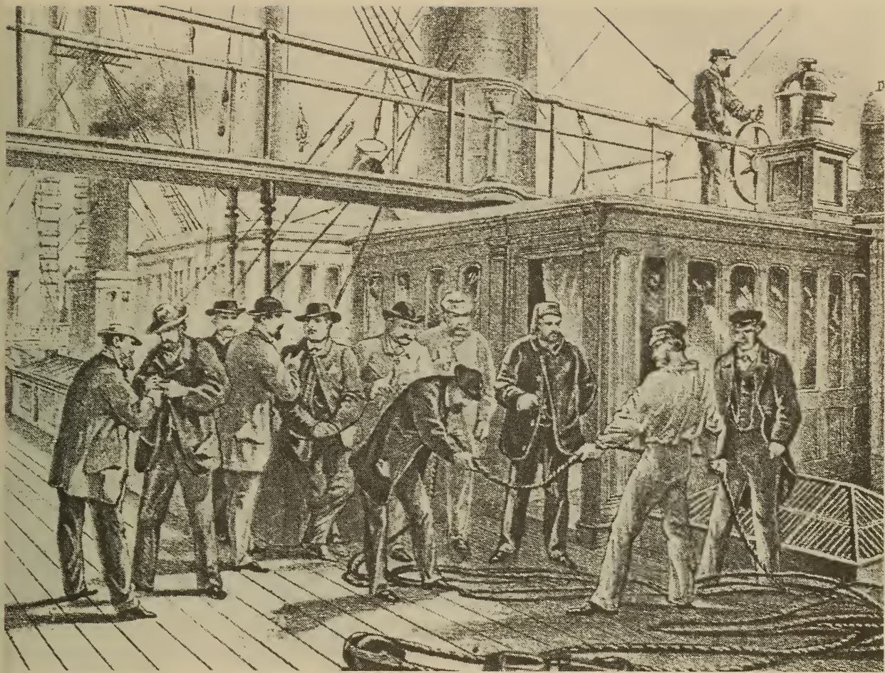
Fig. 6. Searching for fault after recovery of cable from bed of the Atlantic, July 31, 1865 (courtesy Burndy Library).
