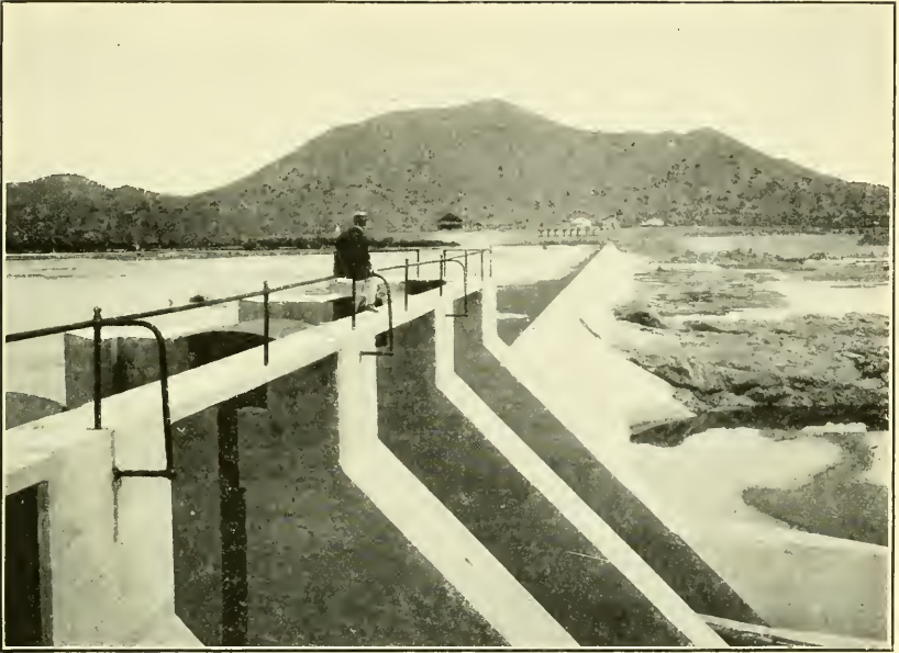
1. GRANITE REEF DAM, SALT RIVER PROJECT.
