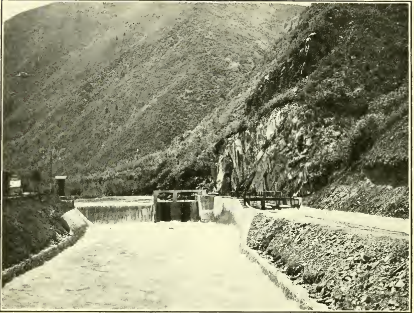
1. DIVERSION DAM, SPANISH FORK RIVER, STRAWBERRY VALLEY PROJECT.
