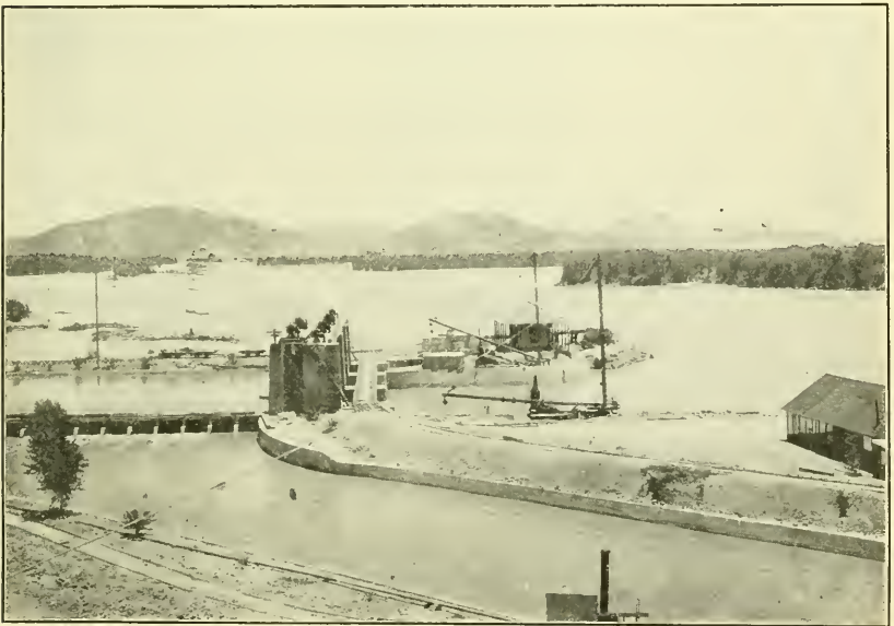
2. LAGUNA DAM, YUMA PROJECT.
