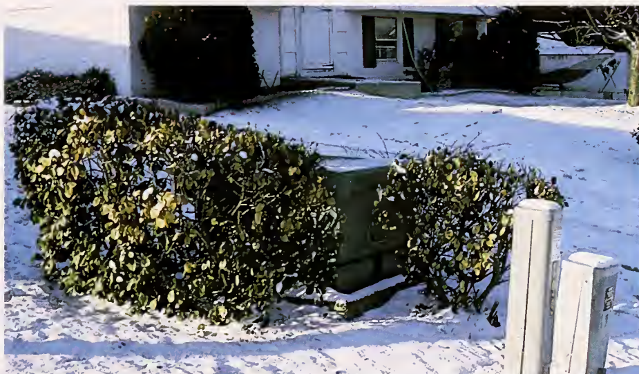
Improperly planted shrubs around underground pad mount transformer can be dangerous to workers in a storm.
