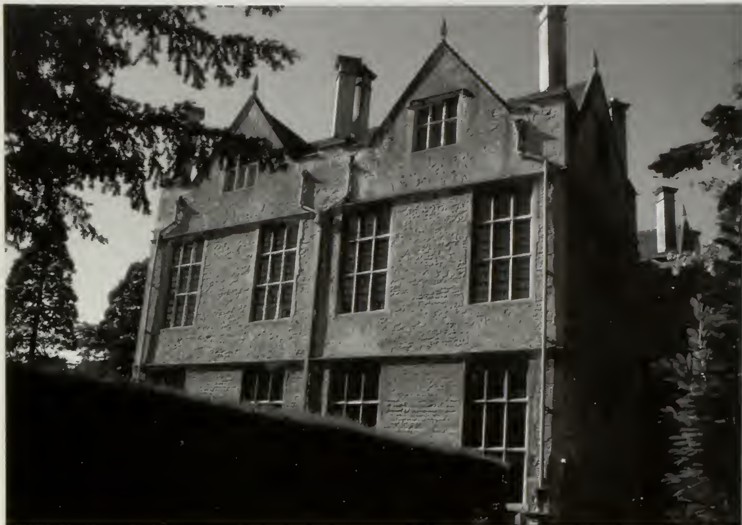
Fig. 5. The east elevation
