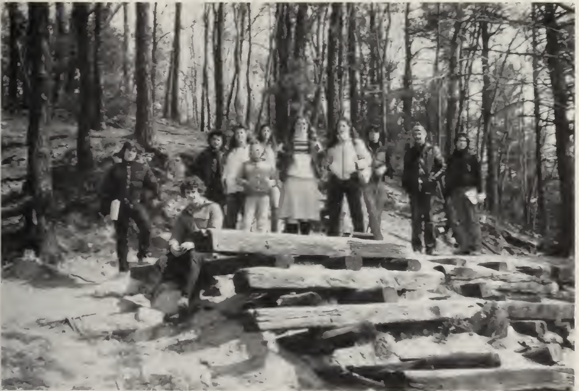
Timber cribbing installed farther along the footpath to arrest erosion of the northern bank of Walden. Photographed on March 20, 1981, by Roland Wells Robbins.
