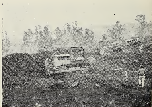
FIG. 5. Bulldozers constructing an earthen barrier in an attempt to keep lava from reaching the Iwasaki camp during the eruption of Kilauea on March 21, 1955.
