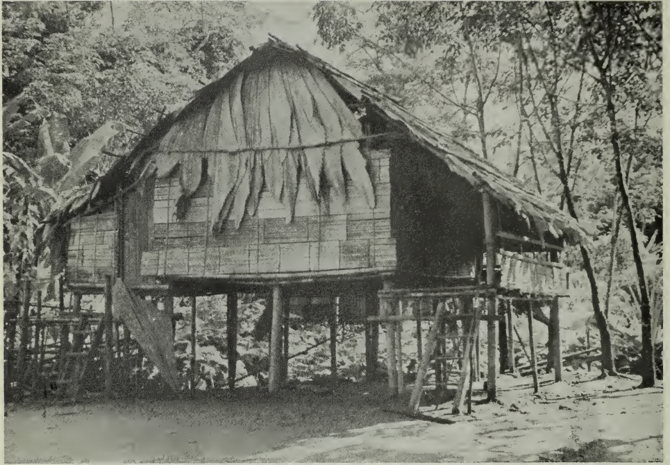
Plate 2. Orang asli house thatched with daun payong Ulu Semenyih, Selangor.
