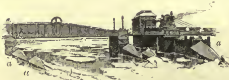
Portion of Bridge over the Yssel, Holland, showing ice-aprons (a, a, a) on the bank and in mid-stream.
