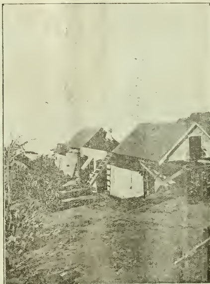
A small Cacao House with sliding roof to admit of the Cacao being quickly protected in case of rain.
