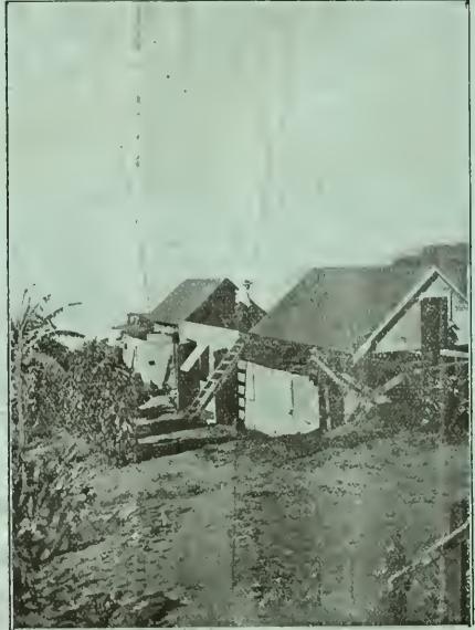
A small Cacao House with sliding roof to admit of the Cacao being quickly protected in case of ruin.
