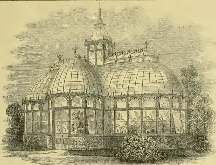
Conservatory erected at Mr. Ley's Nursery, Croydon.
