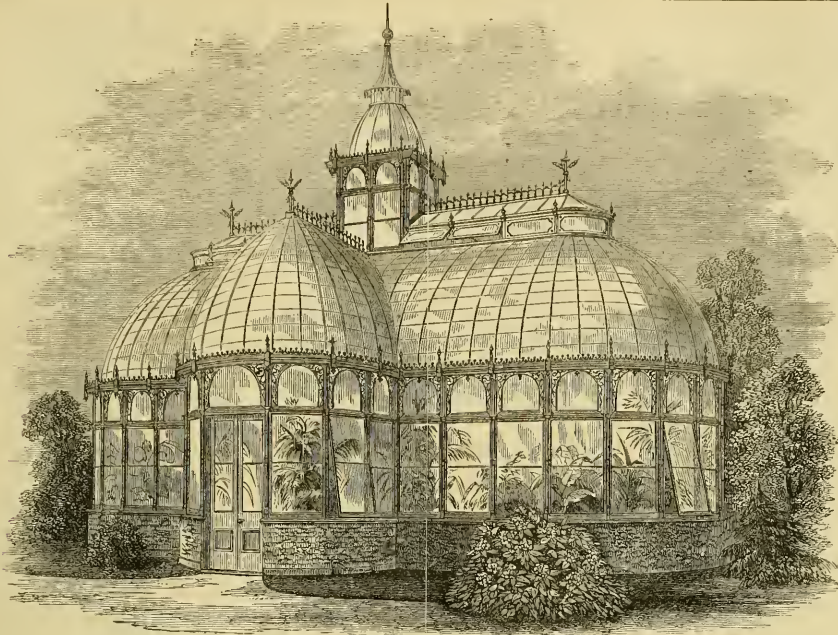
Conservatory erected at Mr. Ley's Nursery, Croydon.
