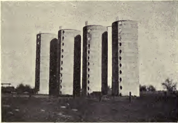
Fig. 31.—Battery of four cement silos on a California cattle ranch. Dimensions 20 feet in diameter, and 46 feet high, capacity about 350 tons each. ( Pacific Rural Press )
