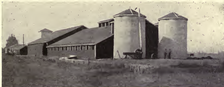
FIG. 29.—A California dairy barn, with concrete silos, accommodating four rows of cows, with a driveway in the middle.
