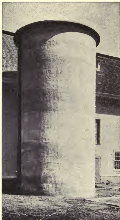
FIG. 28.—A good concrete silo costs more than a wooden silo, but will last indefinitely when properly cared for, and needs no attention beyond an application of a coat of pure cement wash every two or three years. (Wisconsin Station.)
