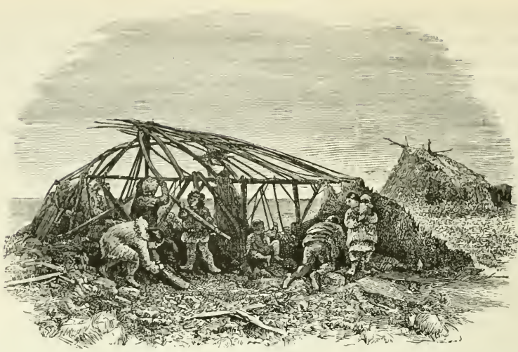
FRAME-WORK OF TCHUKTCHI HOUSE.
