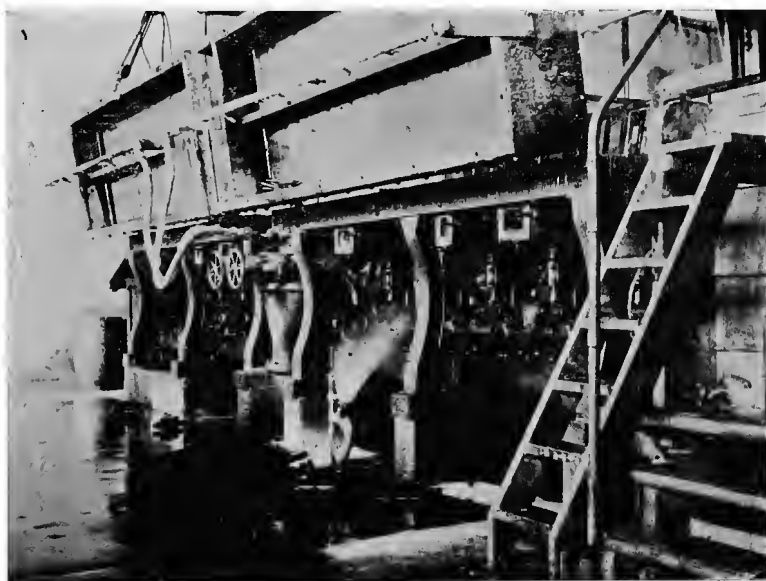
FIG. 10.—Diaphragm plate screen tilted for washing. This screen is located at the head of the paper machine and its function is to screen the paper stock before it passes on to the Fourdrinier wire.
