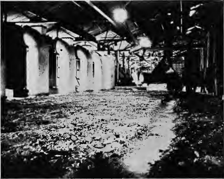
FIG. 61.—Acetate of lime drying over the retorts in the oven house at a large plant at Betula, Pennsylvania.
