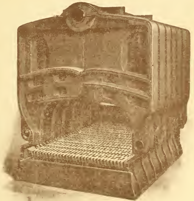
Interior of Sectional Hot-Water Boiler.
