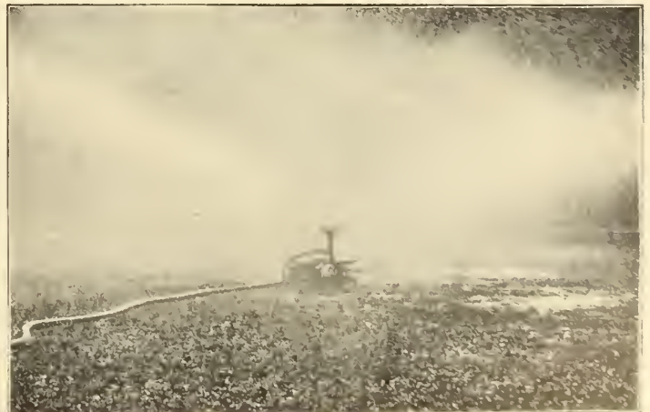
The Park Sprinkler.
