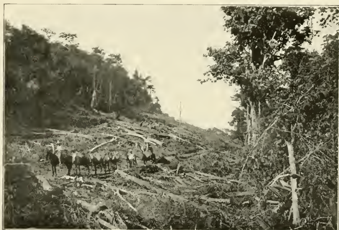
PIECE OF ROAD ON PLANTATION RUILO.
