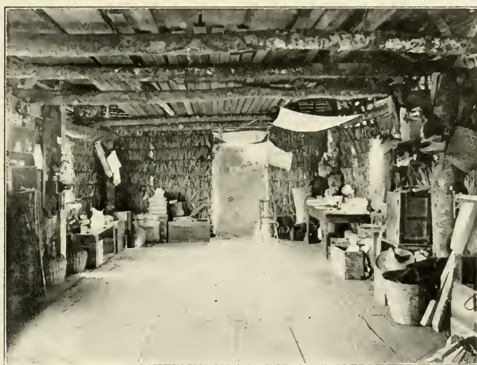
RUBIO.—INTERIOR OF TEMPORARY OFFICE.
