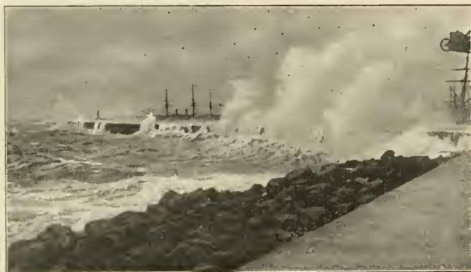
BREAKWATER AT COLOMBO, CEYLON.
