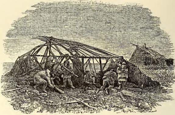
FRAME-WORK OF TCHUKTCHI HOUSE.
