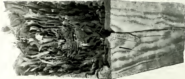
Fig. 2. Part of a tiebeam.
