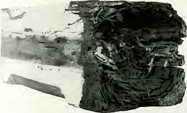
Fig. 3. One end of a pillar.
