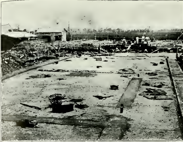
Fig. 1. Construction of a termite-proof concrete layer.
