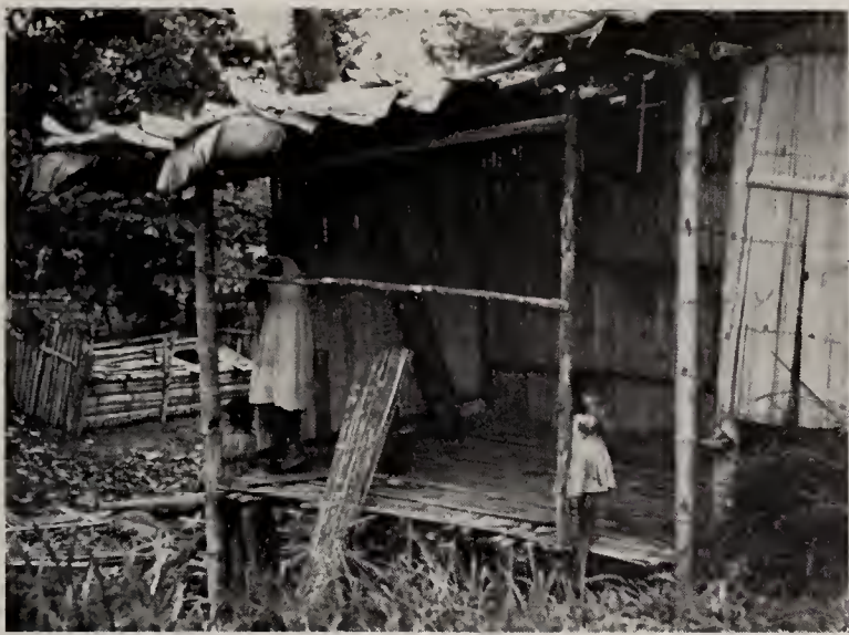
Fig. 16. House under construction in the litoral
