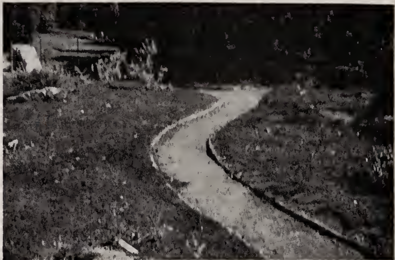
Fig. 2. South section during construction
