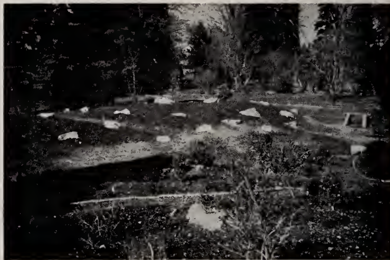
Fig. 5. North section during construction
