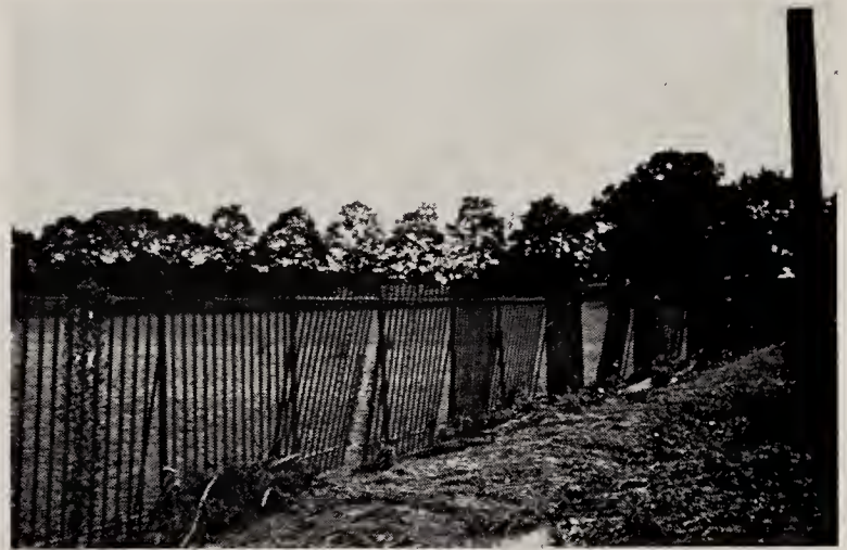
Fig. 84. Damage to Stenton Avenue fence following flood of August, 1955
