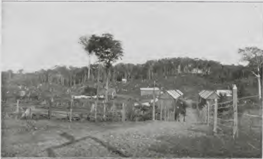
DEL CORTE.—LABORERS CAMP AND CLEARING.
