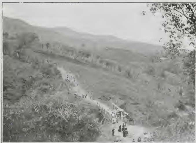
MOUNTAIN ROAD NEAR SAN JOSE.
