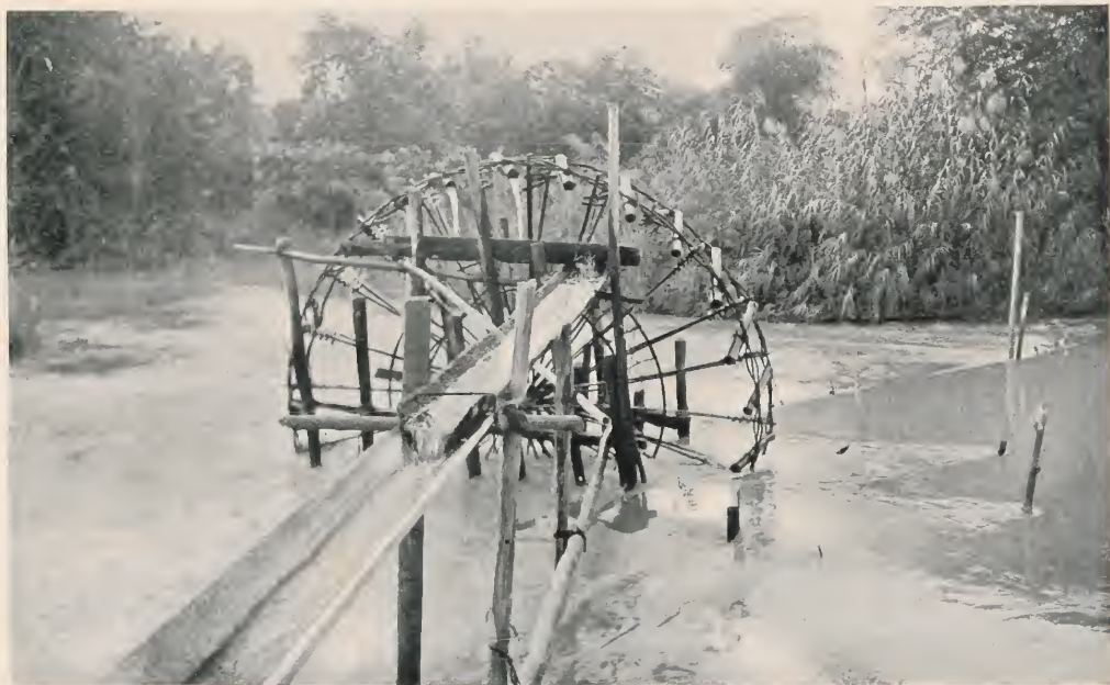
A MALAY WATER-WHEEL FOR IRRIGATING THE RICE FIELDS.
