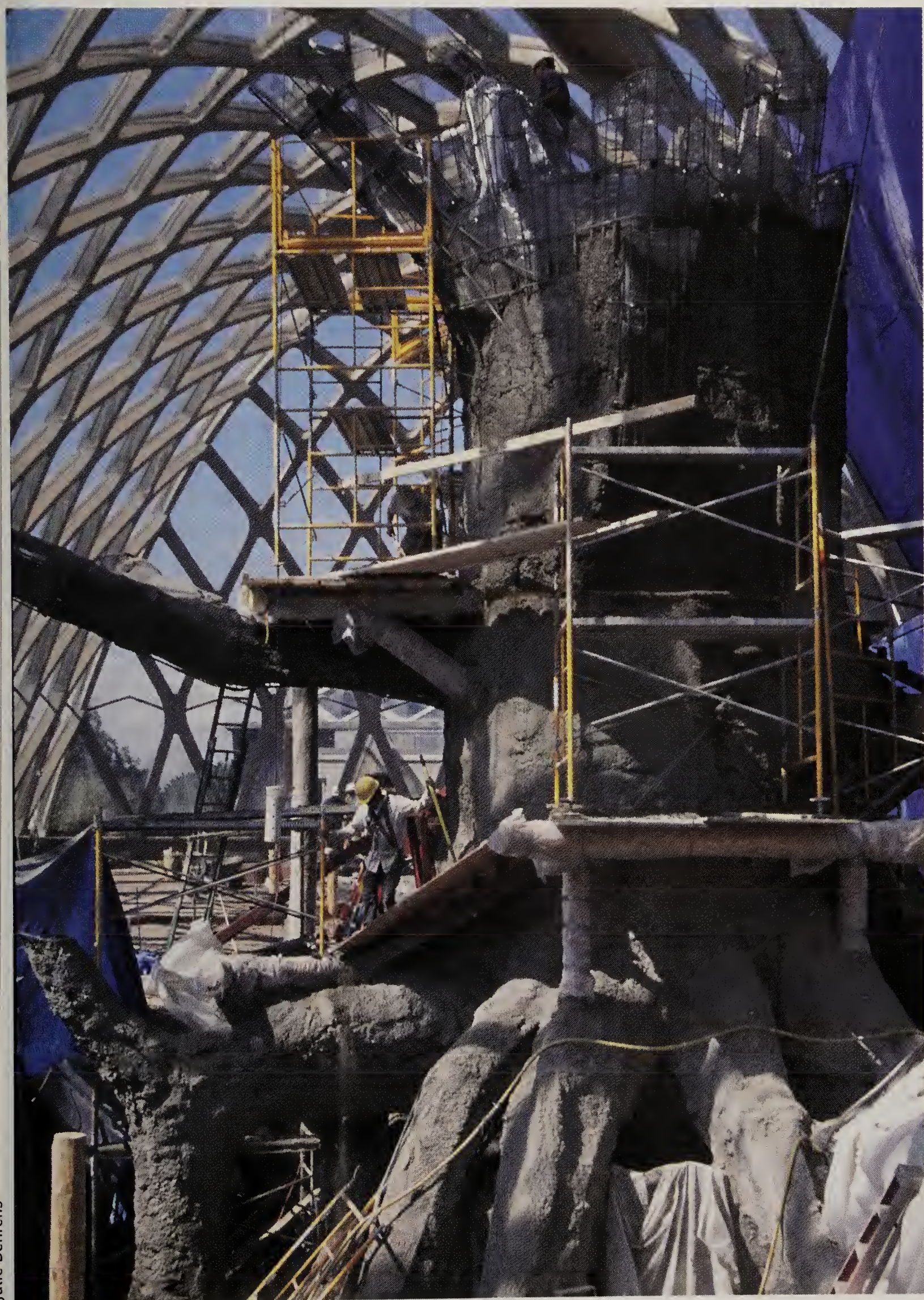
Construction workers finalize the structure of a giant banyan tree — the centerpiece of the new Conservatory plantings.
