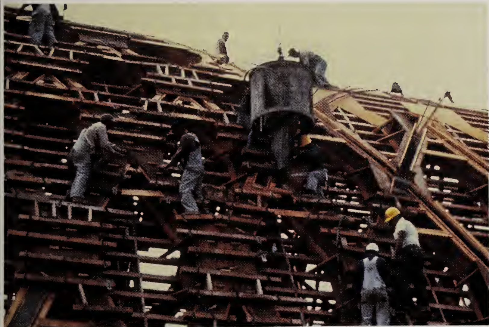
In 1965, workmen pour concrete to form the distinctive domed structure of the Conservatory.
