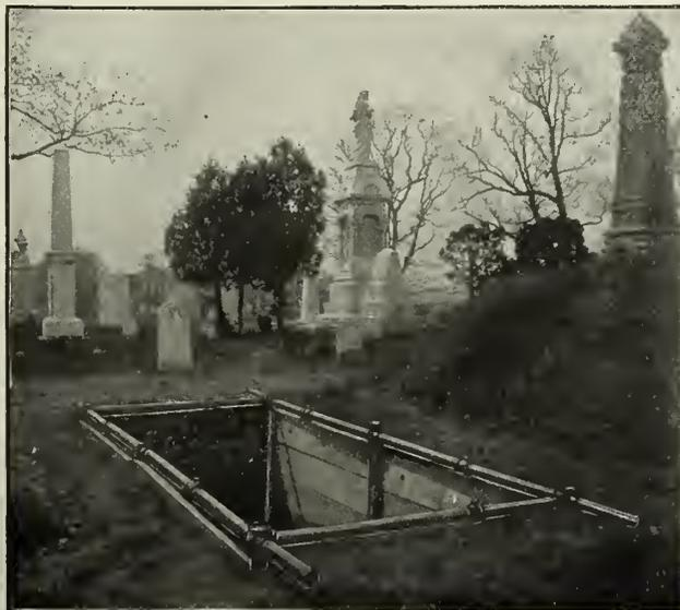
With this device a grave can be excavated in the loosest earth or sand and between other graves without the least danger of caving, no matter how long kept open.
